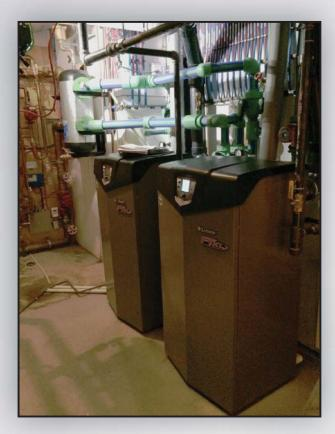
After removing the existing boiler and buffer tank, they installed two 400,000 Btu/hr FTXL Fire Tube Boilers. The FTXL Boilers are equipped with Lochinvar's CON·X·US remote connectivity platform, which allows the homeowner and Byron's Plumbing to monitor and manage boiler functionality from any internet-capable device.
